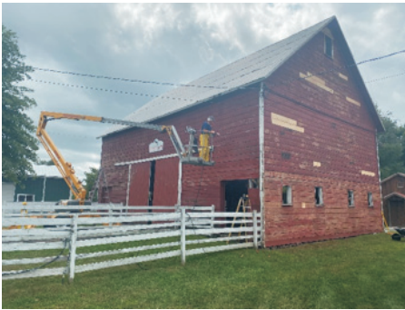
Horse Barn Repair and Painting
